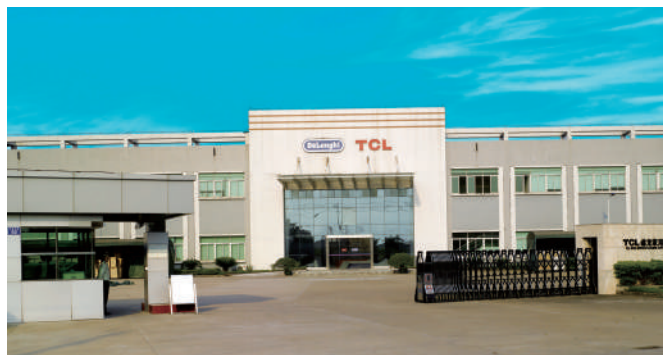
TCL-De' Longhi JV (1 million pcs of portable air-cons & dehumidifiers)
